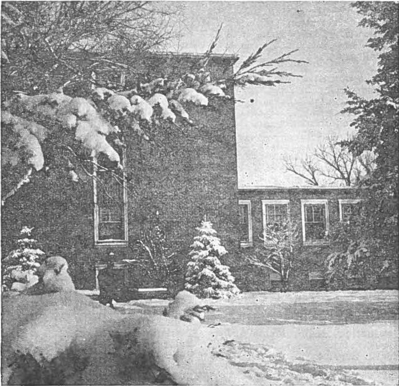
South Entrance to Middlebrook Hall
