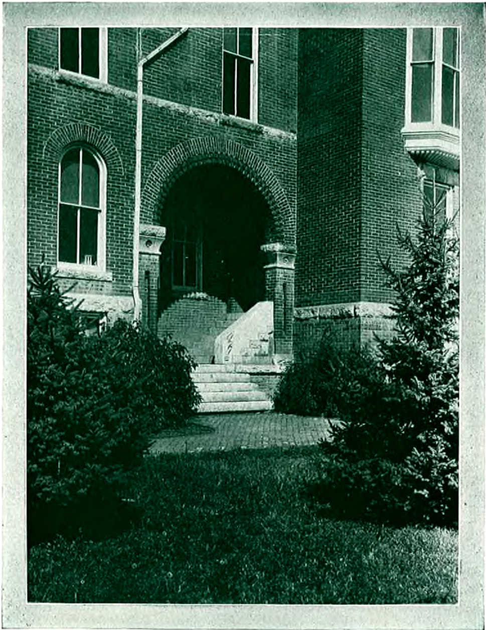
SOUTH ENTRANCE TO THE ADMINISTRATION BUILDING.
