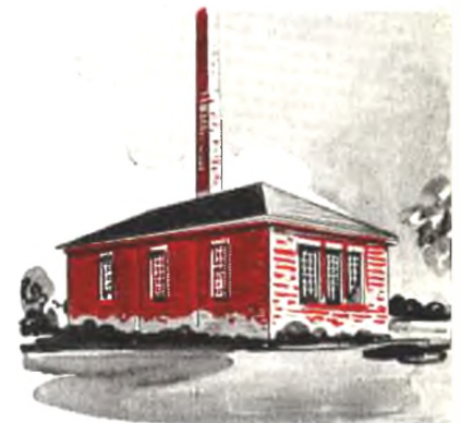
Central Heating Plant
