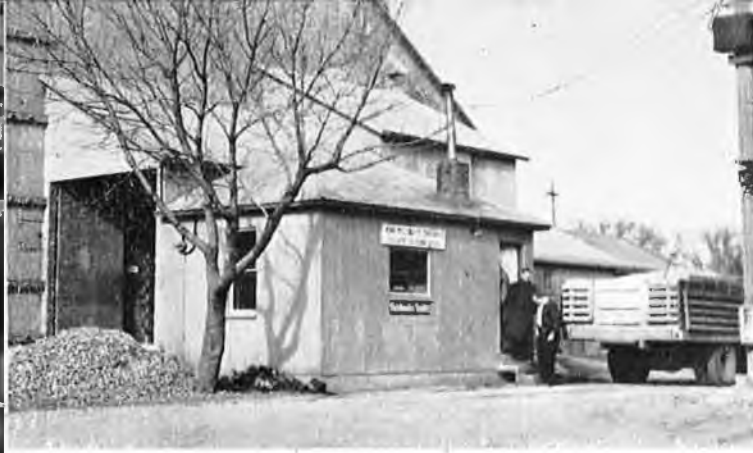
The tall grey bulk of a grain elevator is a prairie landmark. The York Milling and Elevator Company, owner of this elevator, is of service to the entire community with their careful handling of valuable grain products.
