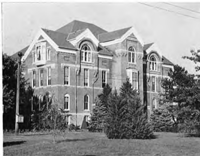
STILL TOWERING over the campus, Old Main sports a renovated roof-top.
