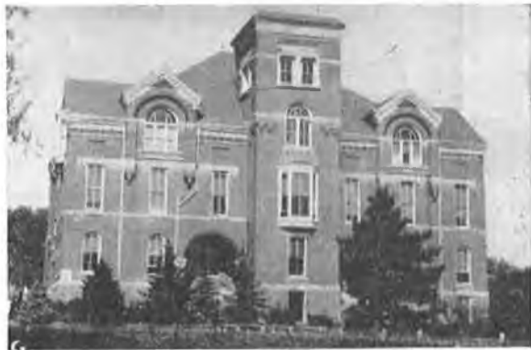
Last week Y. C. started the last quarter of its fiftieth year. Shown above is the Administration Building, southern view.
